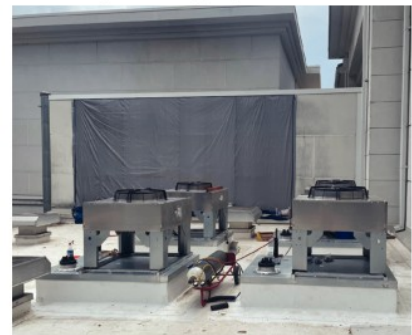
HVAC installation in the works
